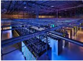
Data Centers Telecomm
